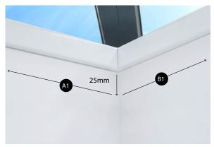
Now measure the Width at the Top, Middle & Bottom of the opening (A). Measure the Length at the far Left & far Right of the opening (B) as indicated. Provide all measurements in MM. Please also indicate if the motor end of the Blind will be situated at either side A1 or A3.
